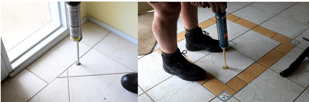
Injecting ARDEX RA56 at left and Dunlop Ardit Crack Filler at right
