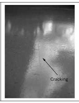
These photos show a cable-heated subfloor in preparation (left) and with a wear surface levelling compound applied (right). The right-hand image shows that the leveling compound has developed linear cracks that mirror the embedded heating cables.
