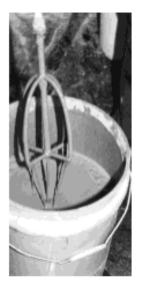
After mixing the smoothing cement should be smooth and free flowing. Note – Do not add water more than the recommended amounts as this can seriously affect the performance of the material.
