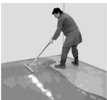
6. The floor spreading tool is used to smooth out the surface after it has been raked or spreading the poured cement if the surface is too irregular to use the thickness rake.
