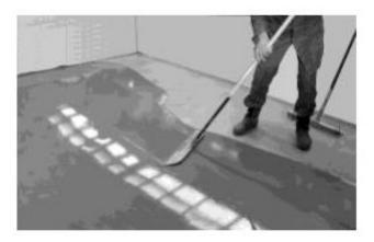
7. The last pass against a door or wall is done by pulling the tool along and walking backwards to the exit point, which is then finished with hand trowels. Note: Do not overwork the material as this causes fines to rise to the surface and results in a soft surface. Also do not work or walk onto material that has been previously laid for more than about 5 minutes.
