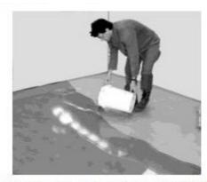
Pour the smoothing cement whilst walking along, and always apply to the wet working edge.
