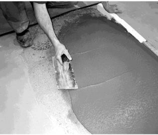
The mixed material is spread to fill the depressed areas, or trowelled into shape to provide falls or form a ramp.
