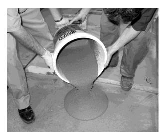
The mixed leveller is applied to the surface by pouring from the mixing container and working to a wet edge.
