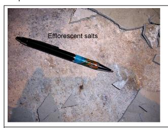
A damp concrete floor treated with a reactive silica-based treatment has developed severe efflorescent salt deposits. The smoothing cement has debonded off the powdery surface.
