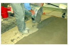
a. The **Minimum** installation thickness for the lightweight topping is **15mm**; however, where a thinner thickness is required, such as filling in slab deflections, neat ARDEX smoothing cements, or ARDEX A45 mortar can be used to provide a smooth transition to adjacent levels.
