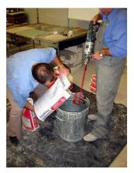
a. When adding the lightweight aggregate, the blades of the "ribbon type " mixing paddle must be visible to ensure that the vortex action of the mixing paddle effectively draws the aggregate (this is particularly important with the SL Grade Polystyrene Bead) into the mortar to blend and coat the aggregate and provide an even distribution throughout the mix.
