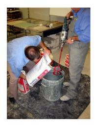
d. When adding the lightweight aggregate the blades of the "ribbon type " mixing paddle must be visible to ensure that the vortex action of the mixing paddle effectively draws the aggregate (this is particularly important with the SL Grade Polystyrene Bead) into the mortar to blend and coat the aggregate and provide even distribution of it throughout the mix.
