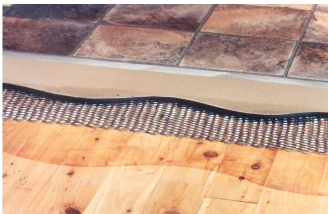
Typical installation over T&G floor.
