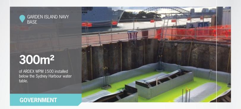
ARDEX was able to provide a solution for below ground works by specifying **ARDEX WPM 1500**. Over 300 square metres of membrane was subsequently applied for this project. **ARDEX WPM 1500** was detailed around pile caps and a "pitch pocket" was created using off-cuts of **ARDEX WPM 1500**. This was then filled with **ARDEX EG 800 F** flowable commercial epoxy grout system and 5/2 aggregate to create a reliable and long lasting waterproofing system.
