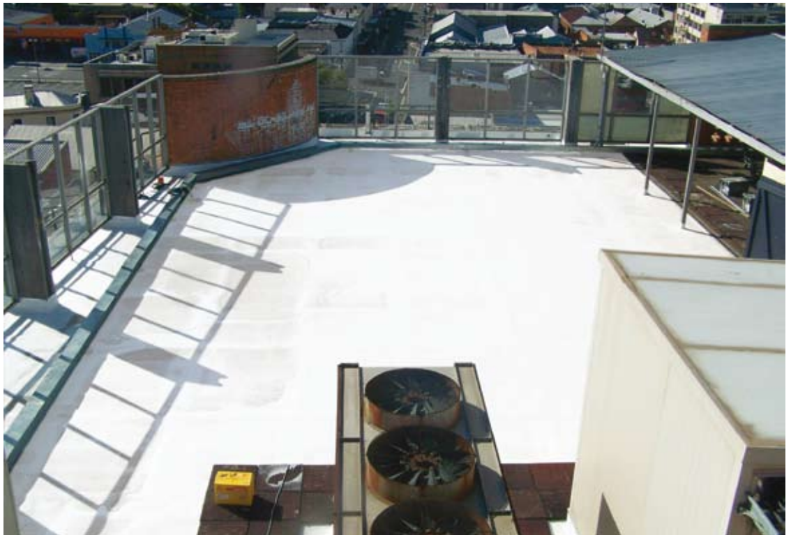
Pictured above: ARDEX TPO installed at the Myer Building in Brisbane Street Mall, Launceston.
