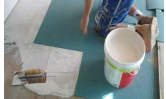
Pictured right: ARDEX DS 40 pre-cut mat installation with AF 266 an indoor and outdoor grass carpet adhesive.
