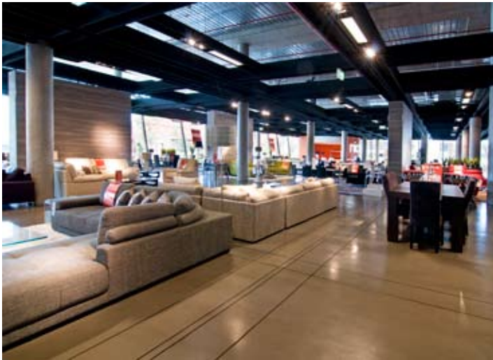
Pictured above: The floor featuring the saw cuts.
