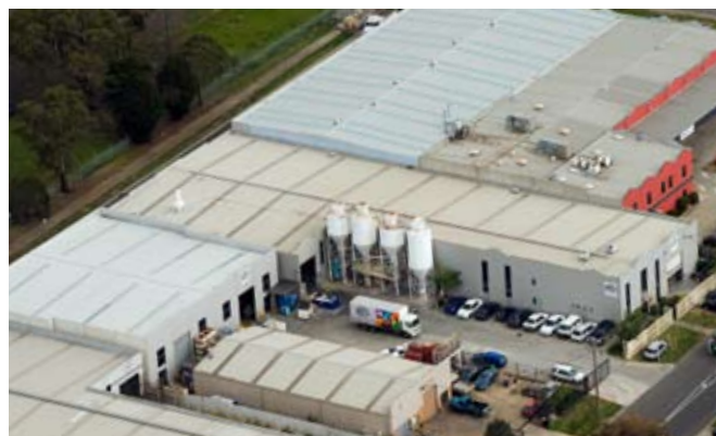
Pictured left: The Ardex Melbourne manufacturing plant. Ardex Australia have manufacturing plants in Sydney, Melbourne, Brisbane, Perth and Adelaide.
