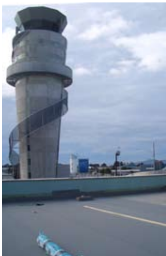
Pictured above: Some of the temporary roofing with the Airport's new communications tower in the background.
