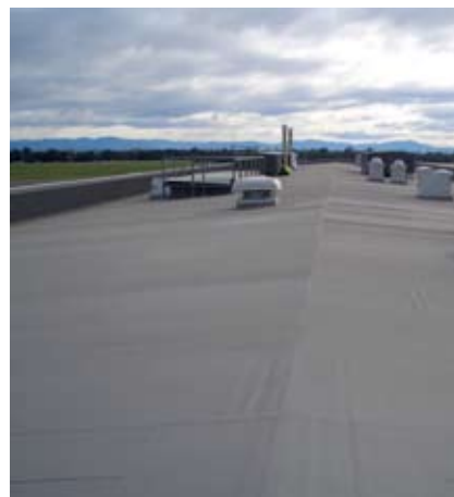
Pictured below: The completed 3000m 2 Butynol roof.
