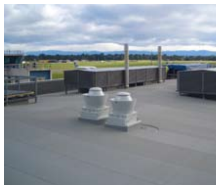
Pictured above: The airport roof required a lot of detailing work.
