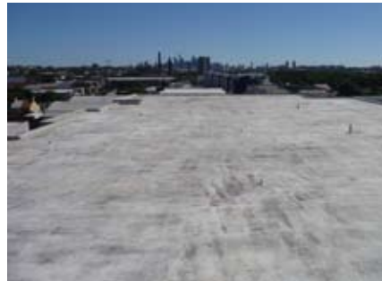
Pictured above: Surface Preparation.
