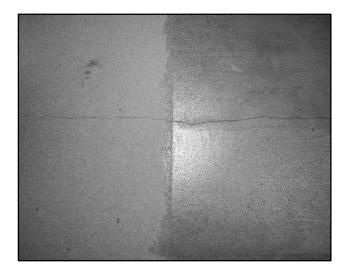
Any marks such as trowel drag marks or changes in colour due to variations in topping colour, texture or water gauging are all brought into sharper contrast when sealed. Again, these features are not visible under normal floor coverings.
