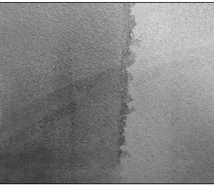
This is a sealed floor which has been subject to over-watering during smoothing cement installation. While this is an attractive swirl pattern, it also highlights softer and weaker areas defined by the white patches. Also, note the sanding marks.
