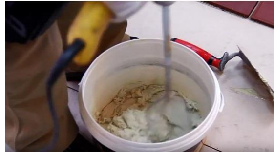
Mixing in the filler powder
