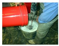
Swirling the mixer around the mixing container assists the distribution of the beads.
