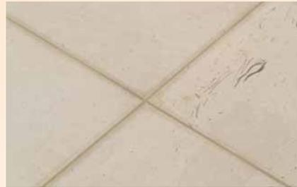
Moisture sensitive natural stones grouted with a traditional cement-based grout, resulting in unsightly water staining at the tile edges.
